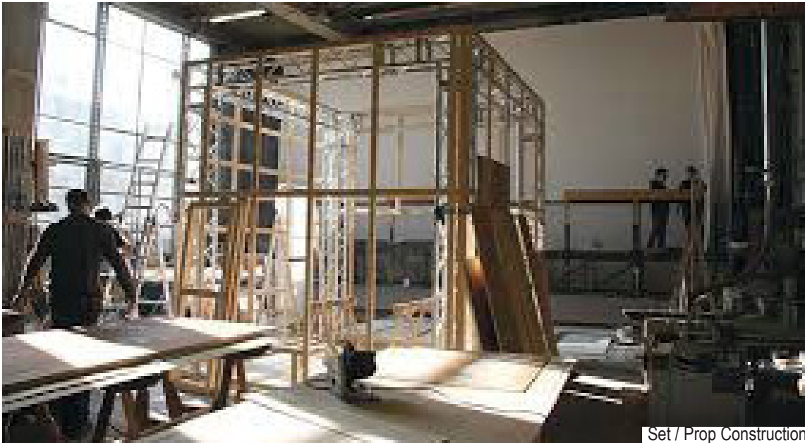
Set / Prop Construction
